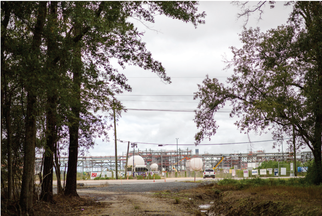
Plant Construction Site #1 - Mossville, October 31, 2018 (COURTNEY DESIREE MORRIS)
